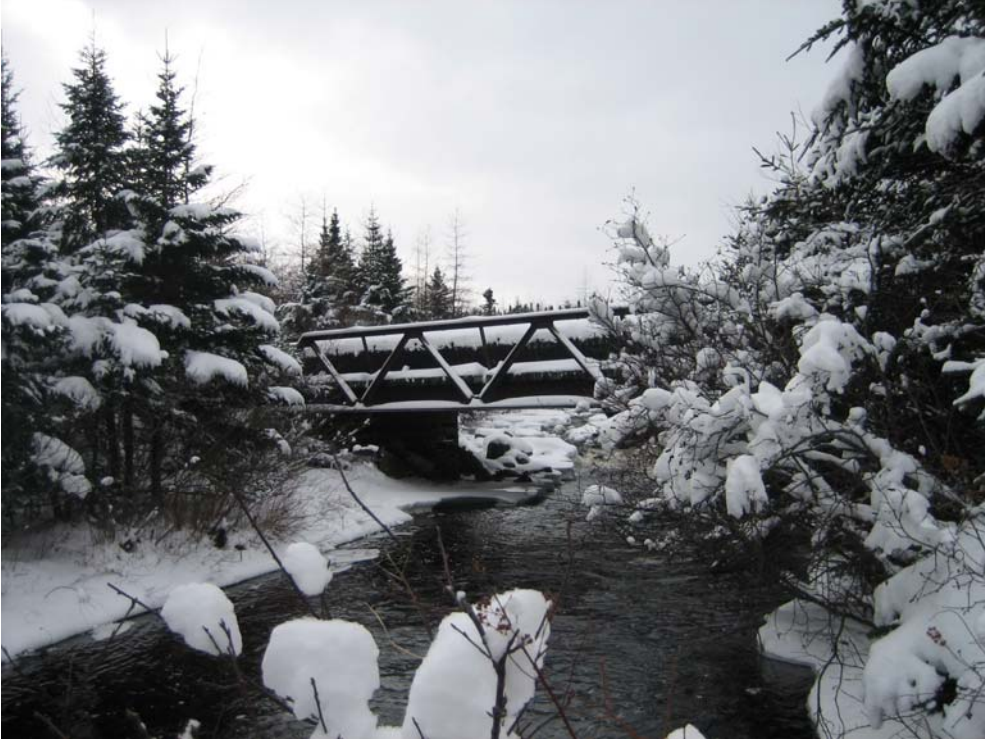
Picture 1: Rattling Brook below Bridge RTWQ Station Location
