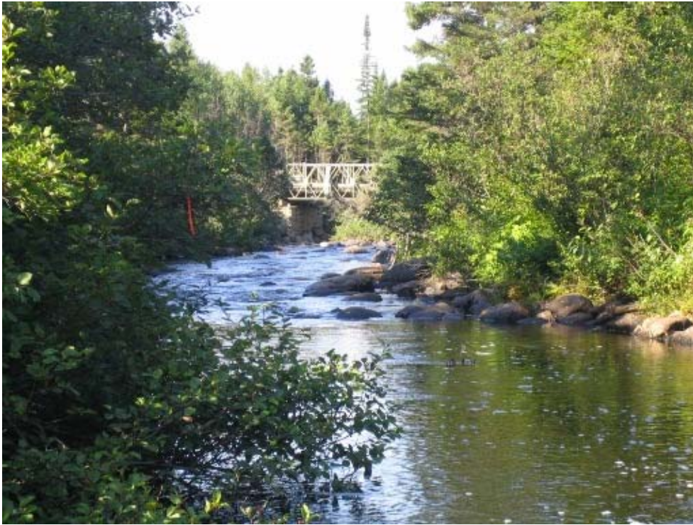
Picture 1: East Pond Brook RTWQ Station Location (looking downstream)
